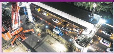
On January 10, 2024, Chennai Metro Rail marked a significant milestone by implementing an innovative puller axle system, which facilitated the transportation and installation of a massive 30m 'U' girder in the Phase 2 project. This project, undertaken by M/s L&T, features the longest 'U' girder span ever achieved in metro rail construction.
