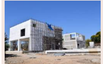
Ancillary building work in progress at Shenoy Nagar Station
