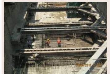
Base slab rebar work in progress at ES-01 at Washerment Station
