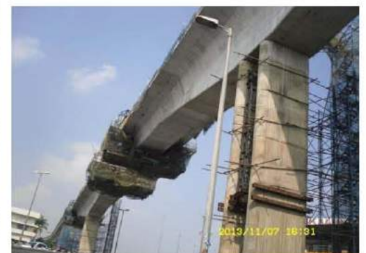
Balanced Cantilever method In-situ casting
