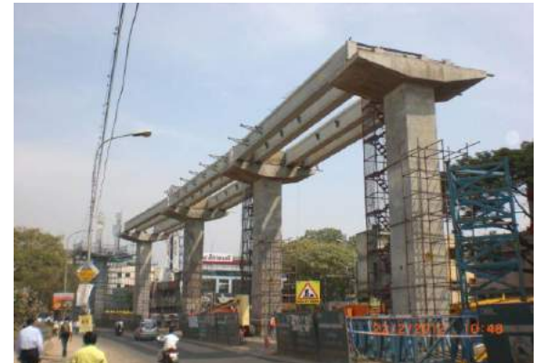
Viaduct spans – I girders erected by Road Crane Method
