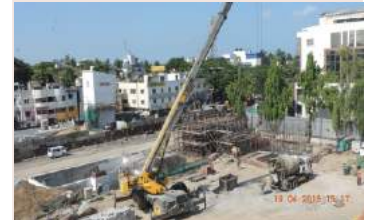
Vent Shaft work in progress at Thirumangalam Station
