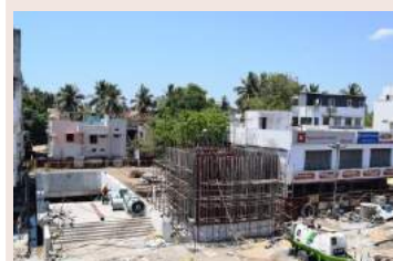
Firemen Staircase work in progress at Anna Nagar East Station
