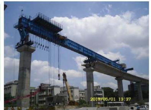
Pre-cast Segments Launching by LG (Launching Girder)
