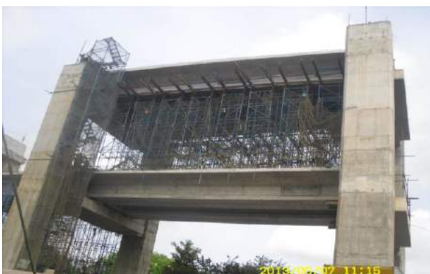
Cast in situ method – Alandur Viaduct
