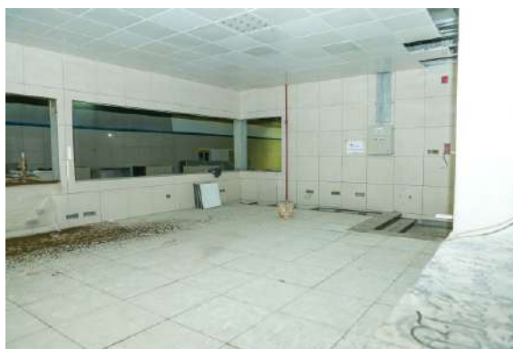
Work in progress at Saidapet Metro Station
