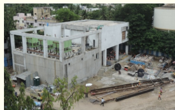
Thirumangalam Metro Station
