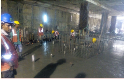
Nandanam Metro Station
