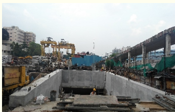
Kilpauk Metro Station
