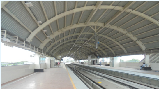
Guindy Metro Station
