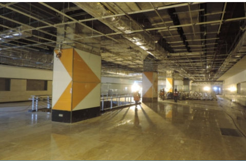
Work in progress at Thirumangalam Metro Station
