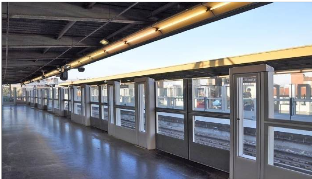
FIGURE 9.9: FULL HEIGHT PSD
