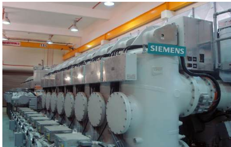
FIGURE 12.1 : GAS INSULATED SWITCHGEAR
