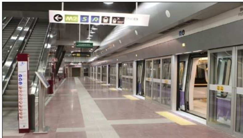
FIGURE 9.5: PLATFORM SCREEN DOOR
