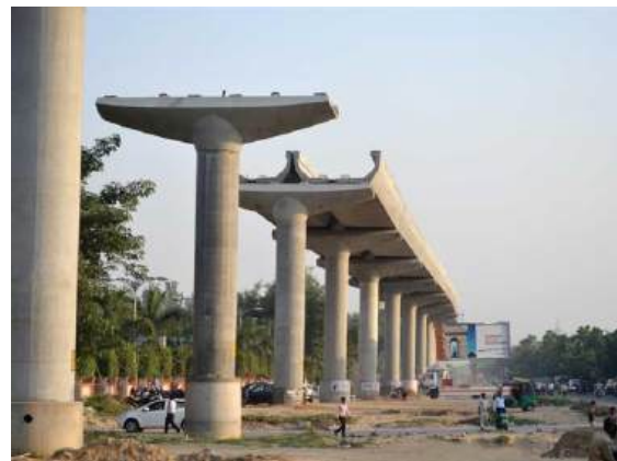
FIGURE 5.39: PRECAST U-CHANNEL SUPERSTRUCTURE
