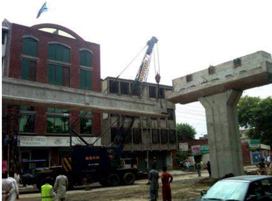
FIGURE 5.41: LAUNCHING OF I-GIRDER
