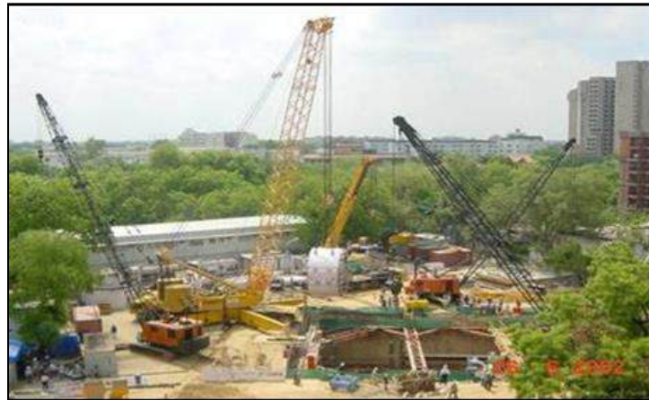
FIGURE 5.50: MAIN SHIELD ERECTION
