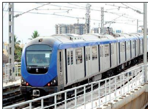
25 kV AC Overhead Catenary System
