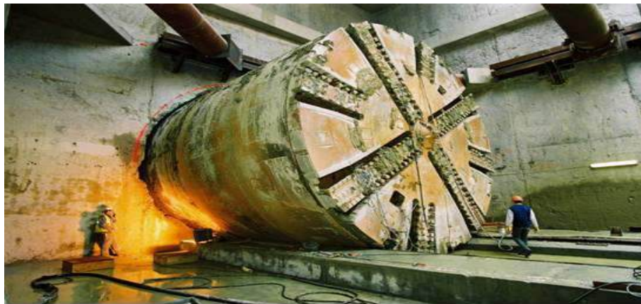
FIGURE 5.53: TBM THROUGH THE DIAPHRAGM WALL
