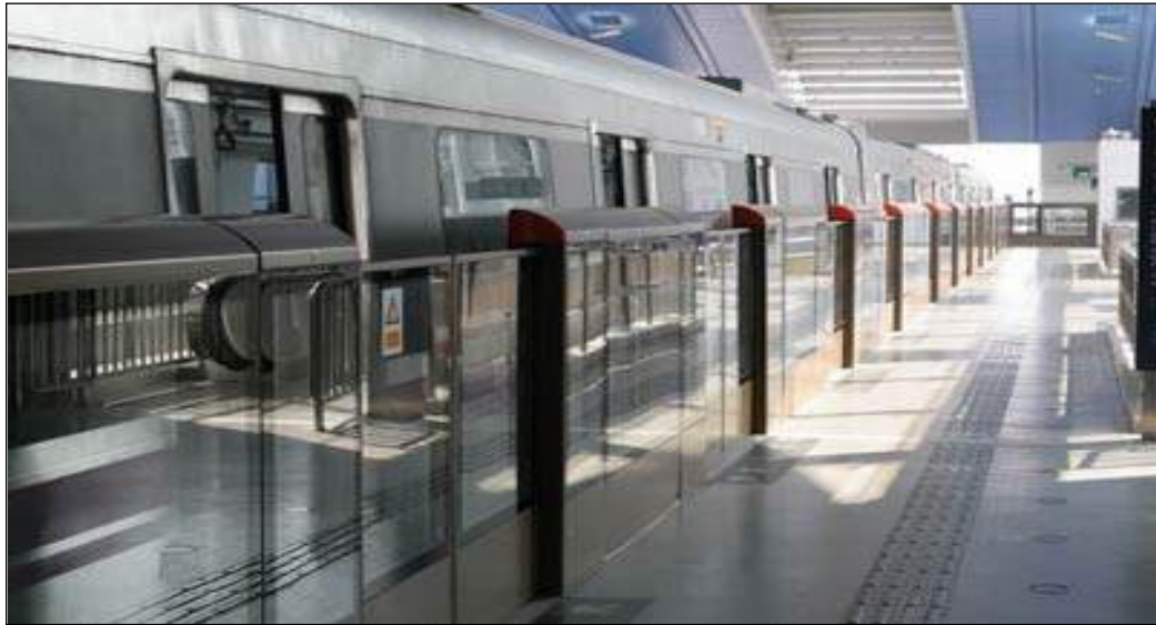
FIGURE 9.9: FULL HEIGHT PSD
