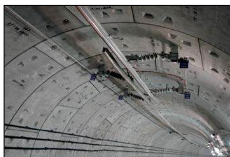
FIGURE 12-3 : 25KV RIGID OHE ARRANGEMENT
