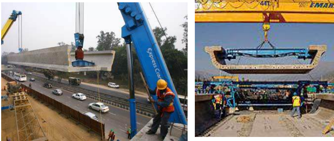
FIGURE 5.40: LAUNCHING OF U-CHANNEL GIRDER
