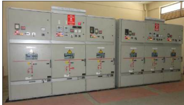
FIGURE 12.2: TYPICAL INDOOR AUXILIARY SUB-STATION (ASS)
