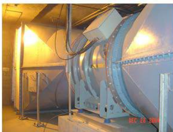
FIGURE 6.13: TUNNEL VENTILATION FAN & DAMPERS
