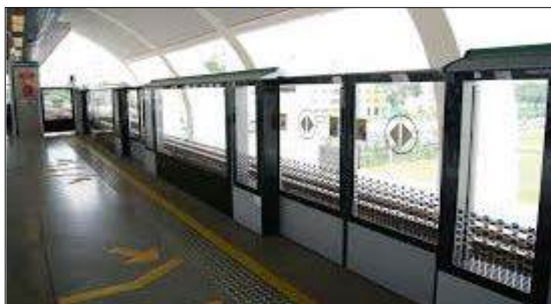
FIGURE 9.6: MANUAL SCREEN DOOR
