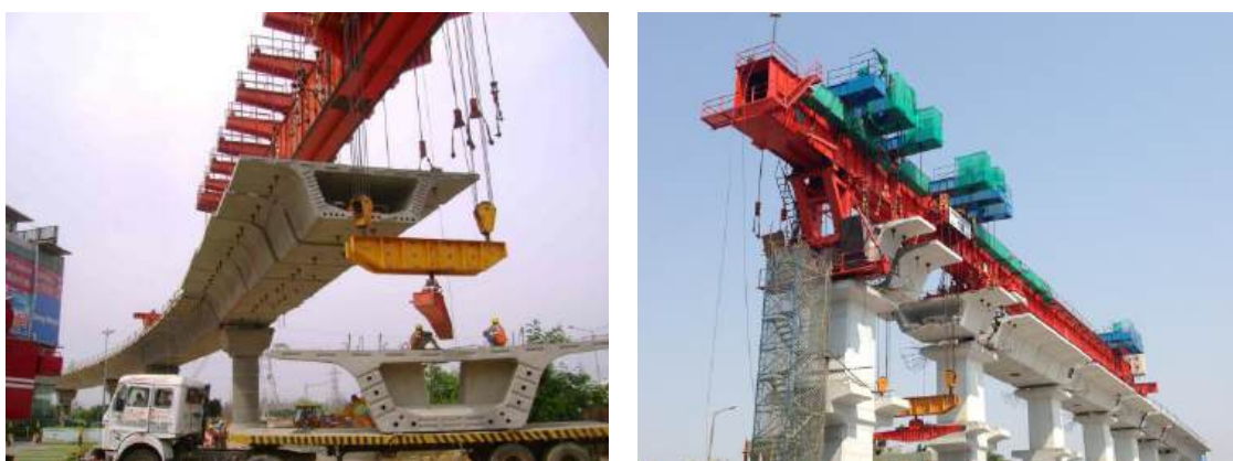
FIGURE 5.38: LAUNCHING OF BOX GIRDER SEGMENTS
