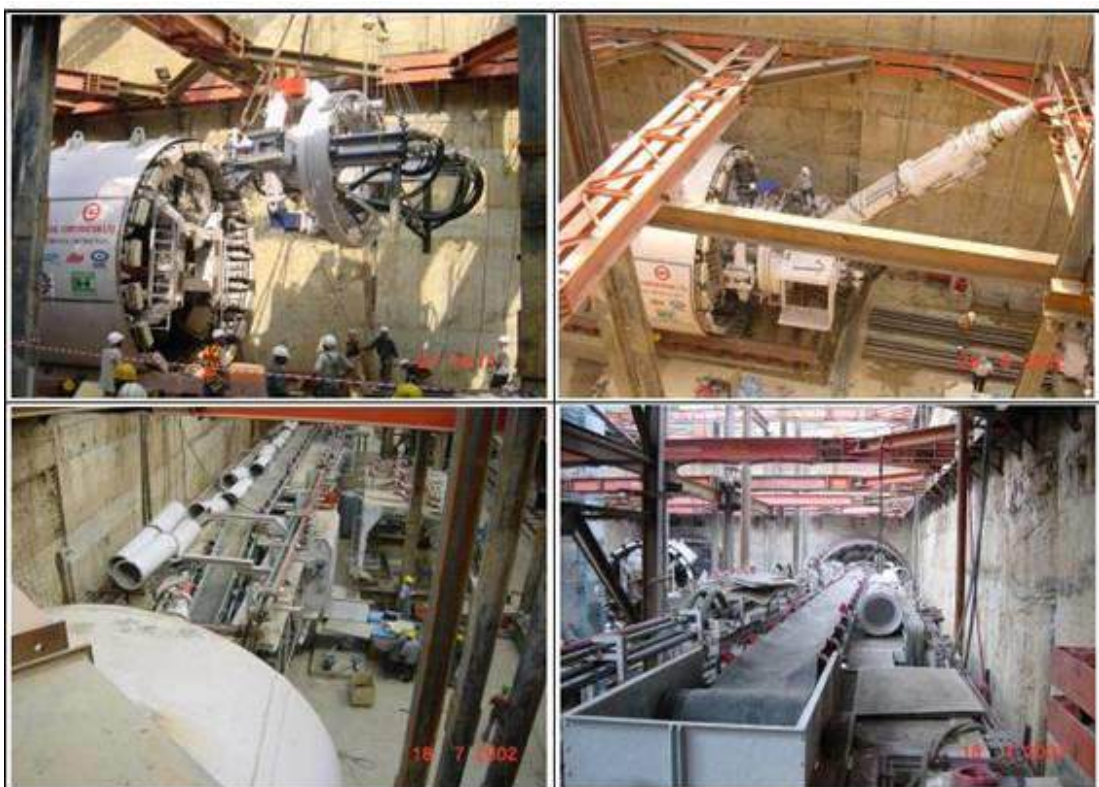
FIGURE 5.49: ERECTOR, SCREW CONVEYOR & BACKUP SYSTEM
