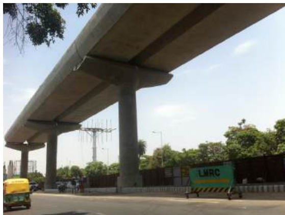
FIGURE 5.39: PRECAST U-CHANNEL SUPERSTRUCTURE
