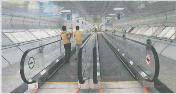
New facility: The travelator connecting both the terminals and the Metro station is ready. ■ G.KRISHNASWAMY
