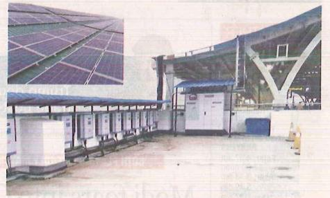
CMRL has successfully installed and commissioned 1120 KWp solar PV power plant in roof top area of two elevated stations, Alandur and St Thomas Mount stations, and in the ground areas at metro rail depot, Koyambedu. They are expected to generate around 1,51,200 units per month and save around ₹69,49,152 per year.
